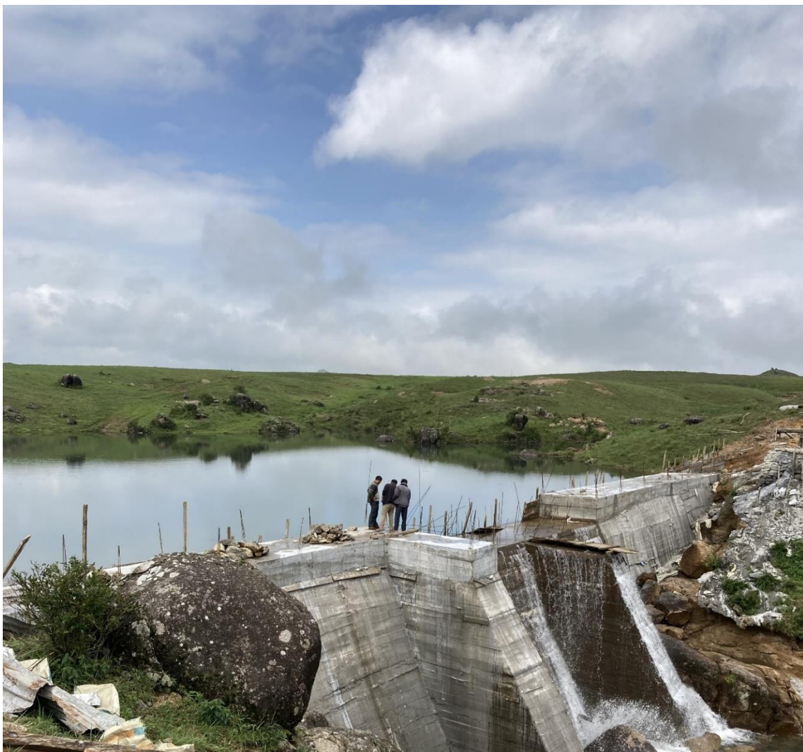
Check Dam at Langsymphut Village
